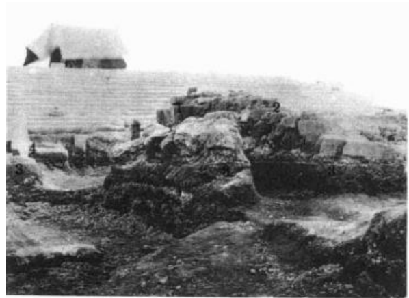
c. Altar, ramp, and floor-level, looking S. Aug. 14, 1908.
